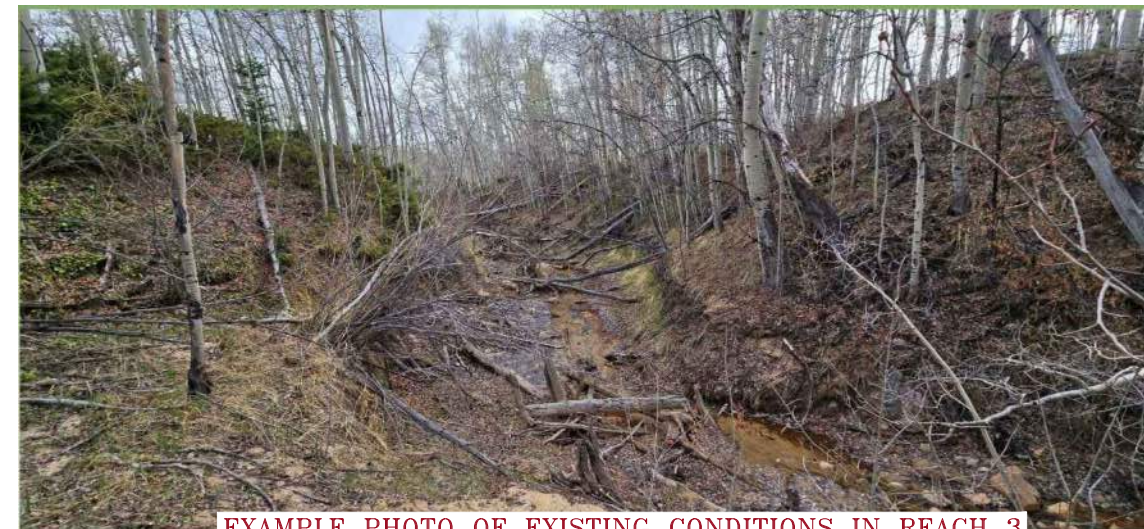
EXAMPLE PHOTO OF EXISTING CONDITIONS IN REACH 3
